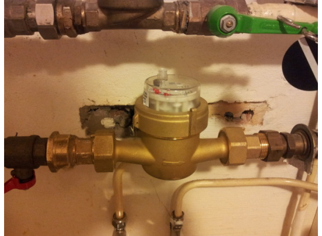
A new water meter with flow measurement capabilities is installed
