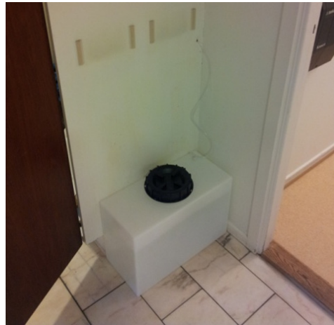
A special Anolyt water tank is fixated
