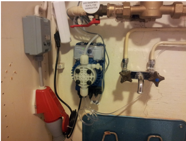
An adjustable water pump is installed
