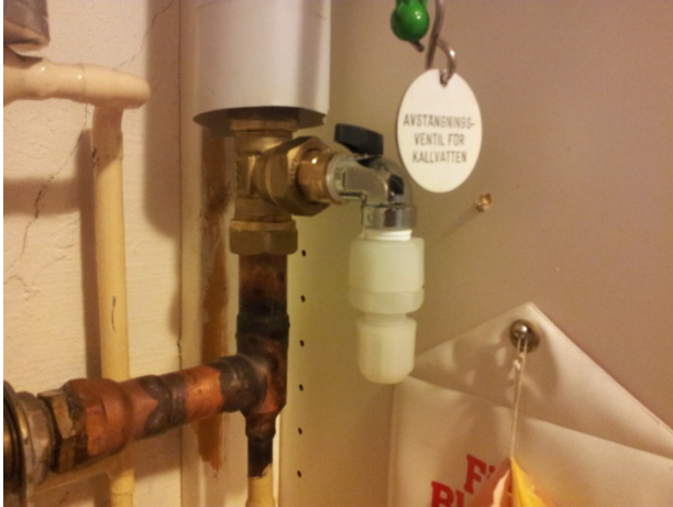
A Ball valve and a pipe connection is fixed to the cold water incoming pipe
